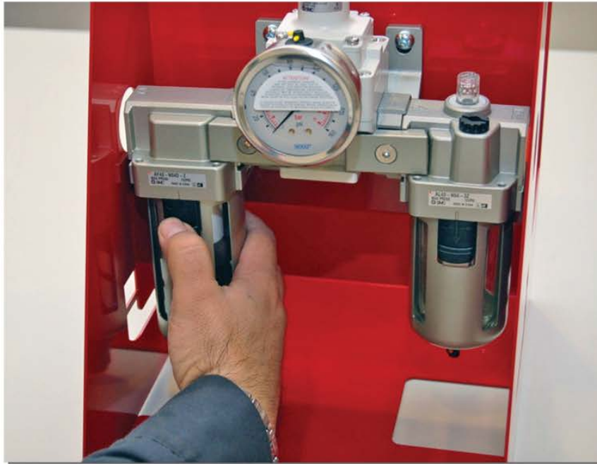
Figure 15. Emptying the FRL Filter Reservoir
